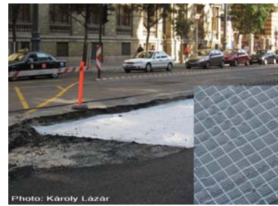
Figure 6. Knitted composite fabric used for driveway reinforcement
