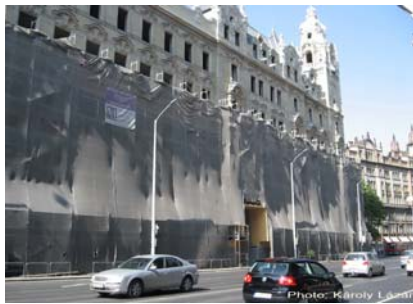
Figure 5. Scaffold covered by raschel net
